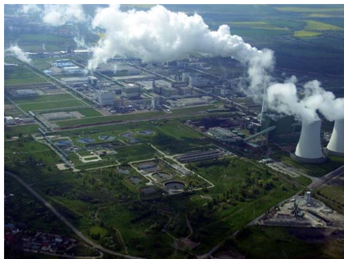
Figure 1. Aerial shot of the DOW Schkopau site, courtesy of Mr. Steffen Bach.
